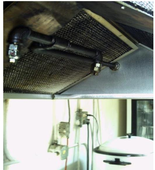
*Obsolete wet chemical 2 piece 1/2 inch nozzles from a pre UL 300 Range Guard system*
