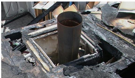
*A fire in this restaurant had nothing to do with the exhaust. The properly installed, double walled duct chase protected the exhaust system.*
