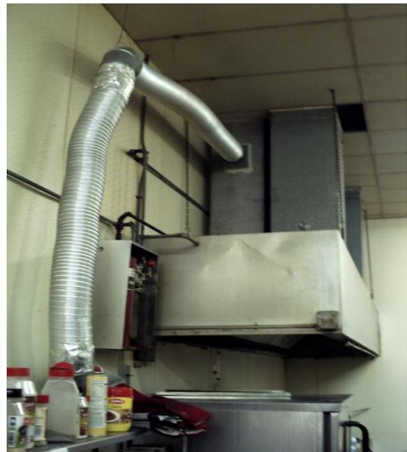
*A rather unbelievable adaptation to the exhaust duct. This material would not last seconds in a fire.*
