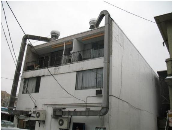
*Two completely unsafe, inaccessible vertical ducts*
