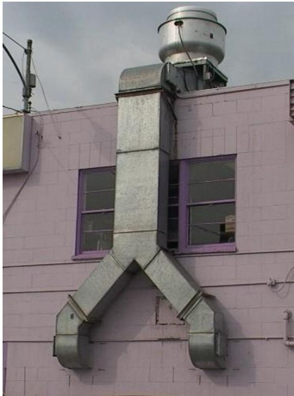
*An exhaust system running up the outside of a building in Anchorage Alaska*
