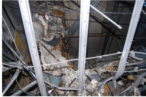
*Duct wrap still connected to the duct above the sub ceiling*
