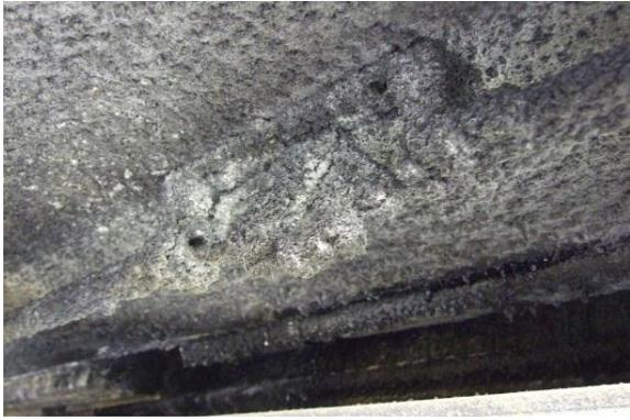
*The fire suppression detector was so covered with grease that it did not activate.*
