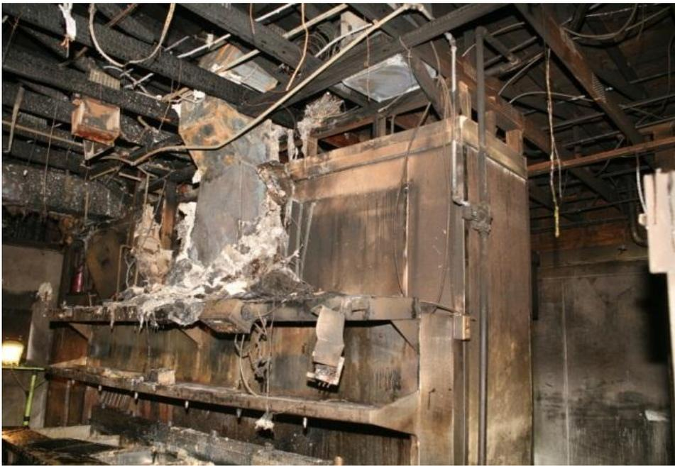
*The fire extended up the duct, radiant heat ignited the 2x4 of the sub ceiling. The duct in the sub ceiling was wrapped but not where the duct was closest to the 2x4s. The wrap collapsed down onto the shelf of the hood.*
