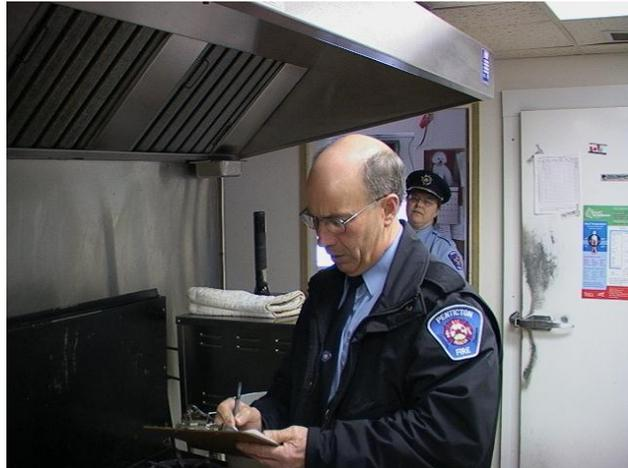
The design/installation phase is the best time to ensure the compatibility of access, balanced fire extinguisher coverage<sup>1</sup>, clearances, tippable fans, and proper air balancing, etc. After the exhaust system is up and running, repairs and upgrades are more difficult.
