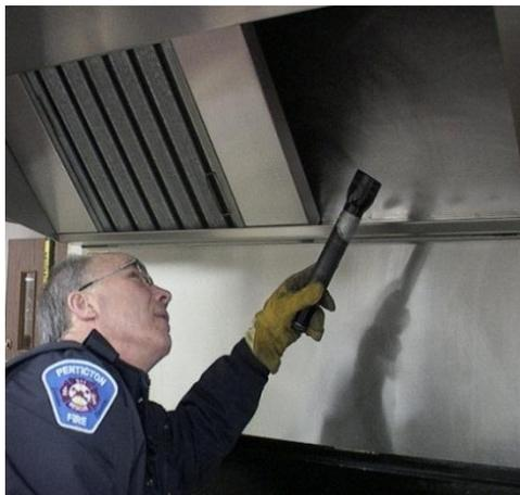
*A Fire Inspector checking behind the filters for grease buildup*
